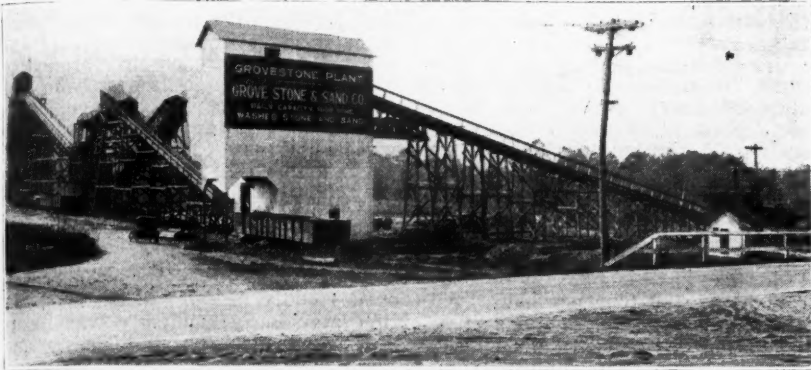
Building in Foreground is For Preliminary Crushing. At the Right is The Incline For the Dump Cars.
